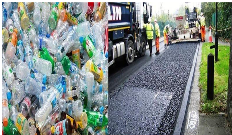
Figure 1.1 Road Constructed from Waste Plastic
